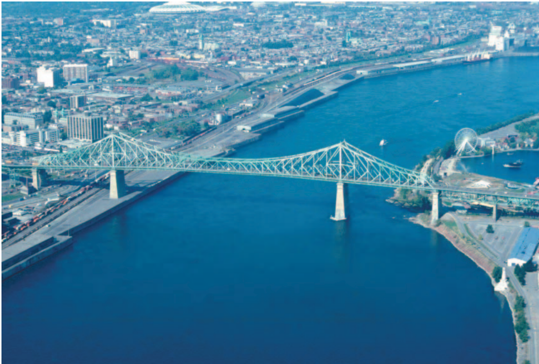
Fig. 3. Jacques Cartier Bridge, Montréal, constructed 1925–1930. When built, the fifth-longest span cantilever bridge in the world with a 1097 ft (334 m) main span (photo taken in October 2000; courtesy of Centre de documentation, Ministère des Transports du Québec, d18881).
