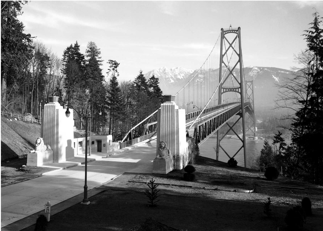
Fig. 5. View looking towards Lions' Gate Bridge, Vancouver, constructed 1937–1938. When erected, the longest-span suspension bridge outside of the United States with a 1550 ft (472 m) main span (photo by Leonard Frank, “View looking Towards Lions' Gate Bridge”, March 1939; courtesy of Vancouver Public Library, VPL 3036).
