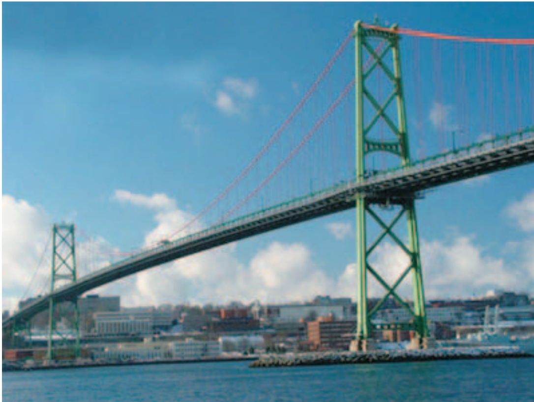
Fig. 6. Angus L. Macdonald Bridge, Halifax, constructed 1952–1955. When erected, the second longest span bridge in the world outside of the United States with a 1447 ft (448 m) main span (photo taken in 2000; courtesy of Cherubini Metal Works Ltd., Dartmouth, Nova Scotia).
