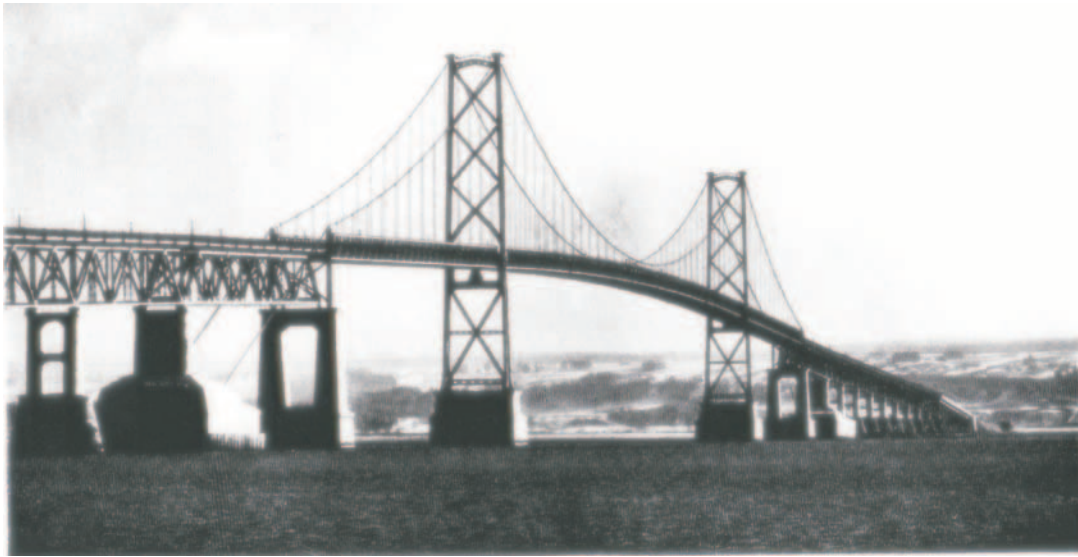
Fig. 4. Île d'Orléans Bridge, Quebec, constructed 1931–1935. An innovative suspension bridge with a 1059' (323 m) main span (photo from the Journal of the Institute of Civil Engineers, October 1936, No. 8, p. 409).
