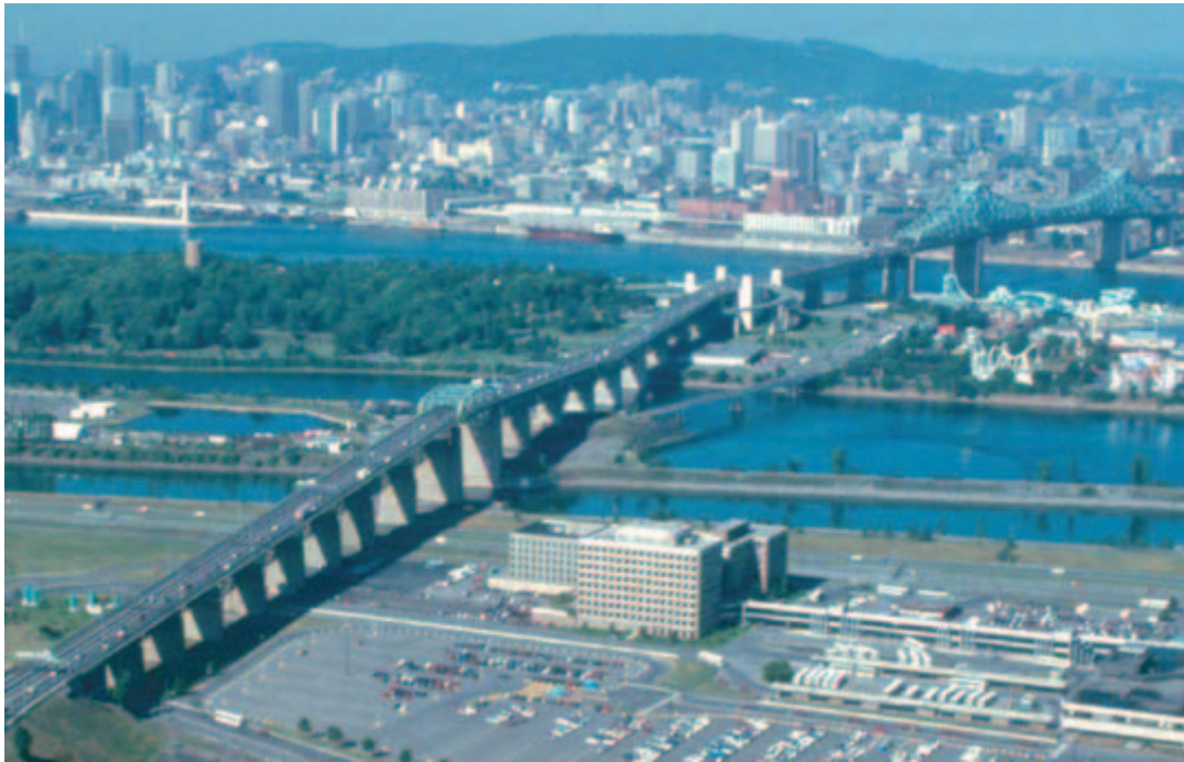
Fig. 8. Raised Seaway section, constructed 1957–1958, of the Jacques Cartier Bridge. At the time, the largest jacking operation anywhere in the world (photo taken August 1991; courtesy of Centre de documentation, Ministère des Transports du Québec, d27465).
