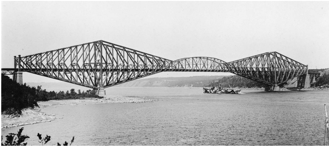
Fig. 2. Québec Bridge, Quebec, constructed 1911–1917. The world’s longest span cantilever bridge with a 1800 ft (549 m) main span (photo by Eugene Micheal Finn, July 1918; courtesy of Library and Archives Canada, Dominion Bridge Company fonds, PA-148584).
